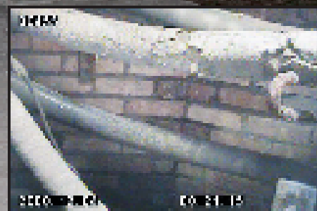
Video still of inside electrical utility vault.
