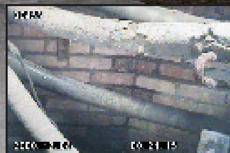
Video still of inside electrical utility vault.
