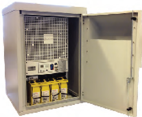
Control enclosure in rack
