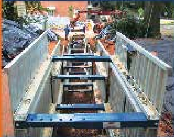
Aluminum Trench Shields
