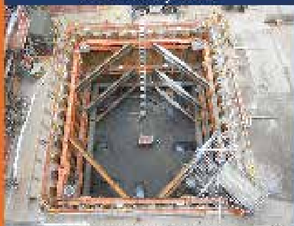
MO Sheeting and Bracing
