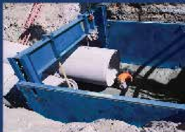
Steel Trench Shields
