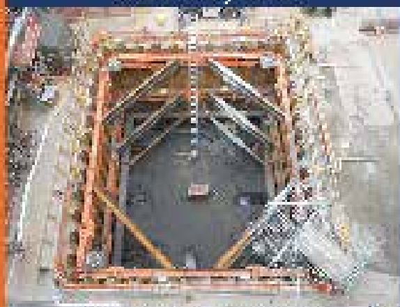
MO Sheeting and Bracing
