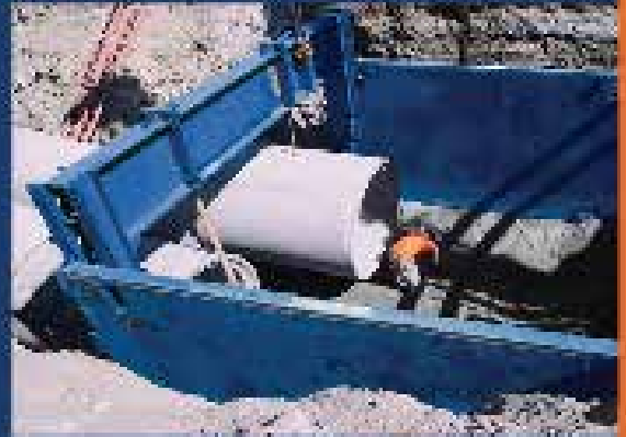
Steel Trench Shields
