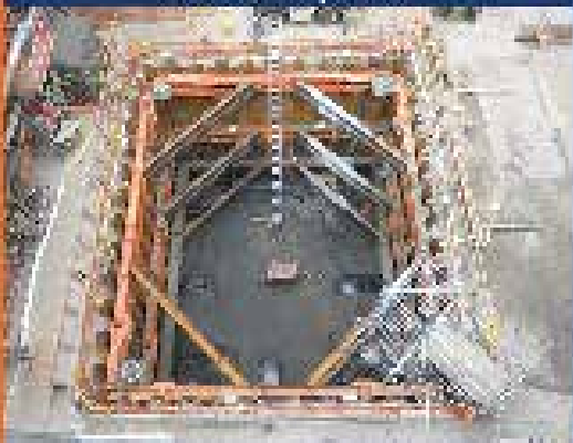
MD Sheeting and Bracing
