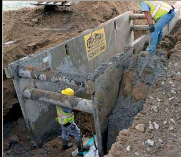
Steel Trench Shields
