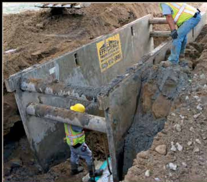
Steel Trench Shields
