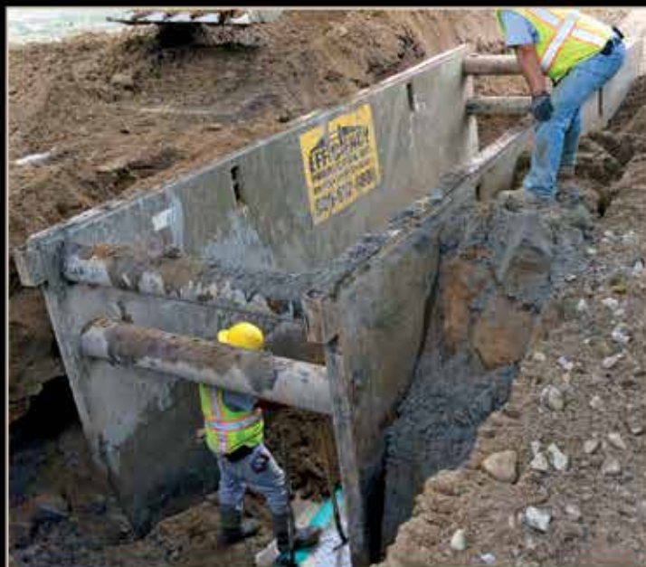
Steel Trench Shields
