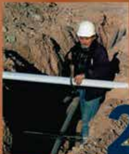
2 Step 2: Cut Split Duct Conduit to Fit
