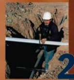
Step 2: Cut Split Duct Conduit to Fit
