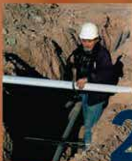
Step 2: Cut Split Duct Conduit to Fit
