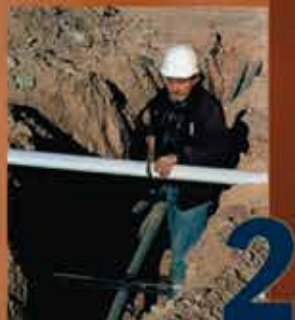
Step 2: Cut Split Duct Conduit to Fit
