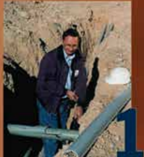
Step 1: Remove Damaged Conduit
