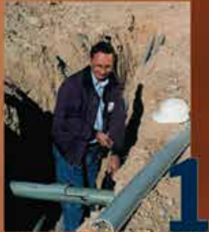
Step 1: Remove Damaged Conduit
