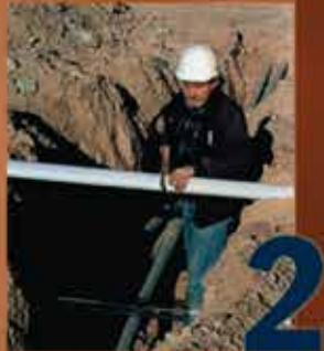
Step 2: Cut Split Duct Conduit to Fit
