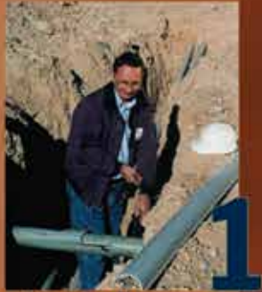
Step 1: Remove Damaged Conduit
