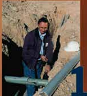
1 Step 1: Remove Damaged Conduit
