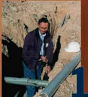
1 Step 1: Remove Damaged Conduit
