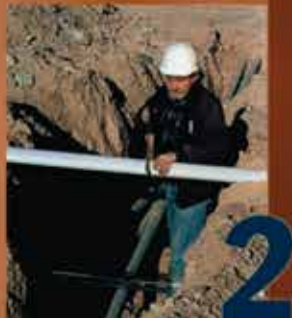
2 Step 2: Cut Split Duct Conduit to Fit
