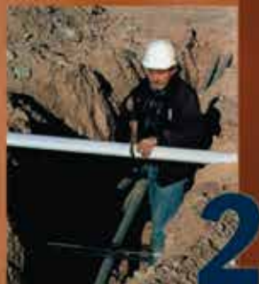
2 Step 2: Cut Split Duct Conduit to Fit
