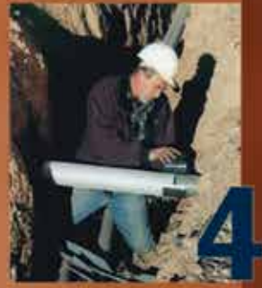
4 Step 4: Attach Adapters
